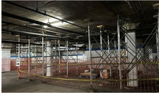
Temporary structural support to keep the upper level from failing.
